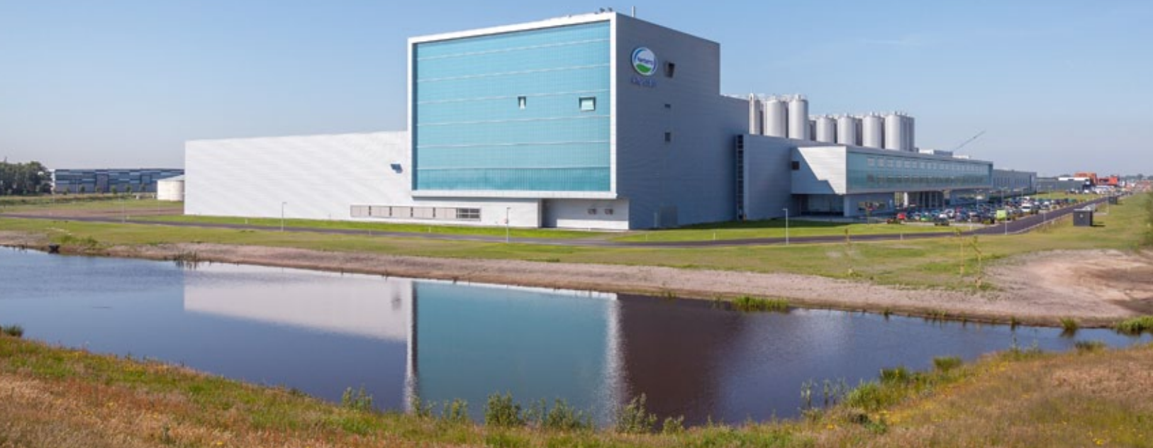
Fonterra's Heerenveen plant has a peak processing capacity of 2.7 million litres of whey per day (photo: Rockwell Automation)
